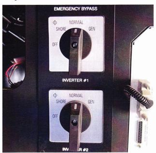
6. Turn on 110 volt breakers as necessary, not to exceed 50 amps for Shore Power or 60 amps for Generator power.
